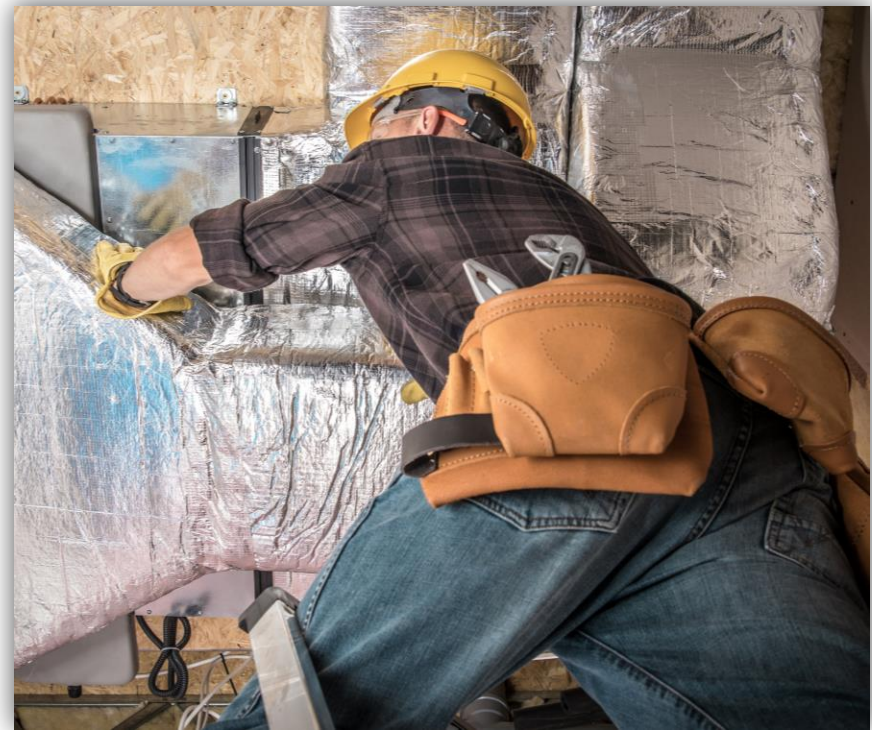
Image: Duct insulation installation
