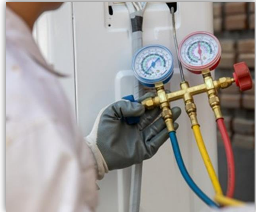
Image: Refrigerant charge verification testing
