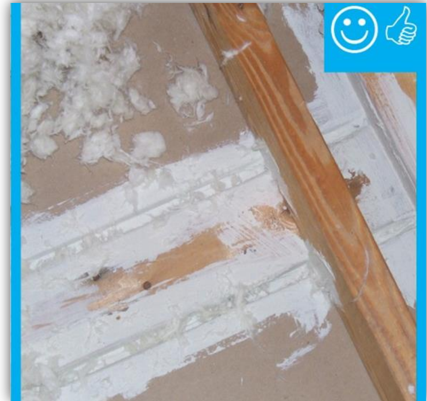
Image: Caulking sealing the drywall and top plate. Courtesy of Building America Solutions Center
