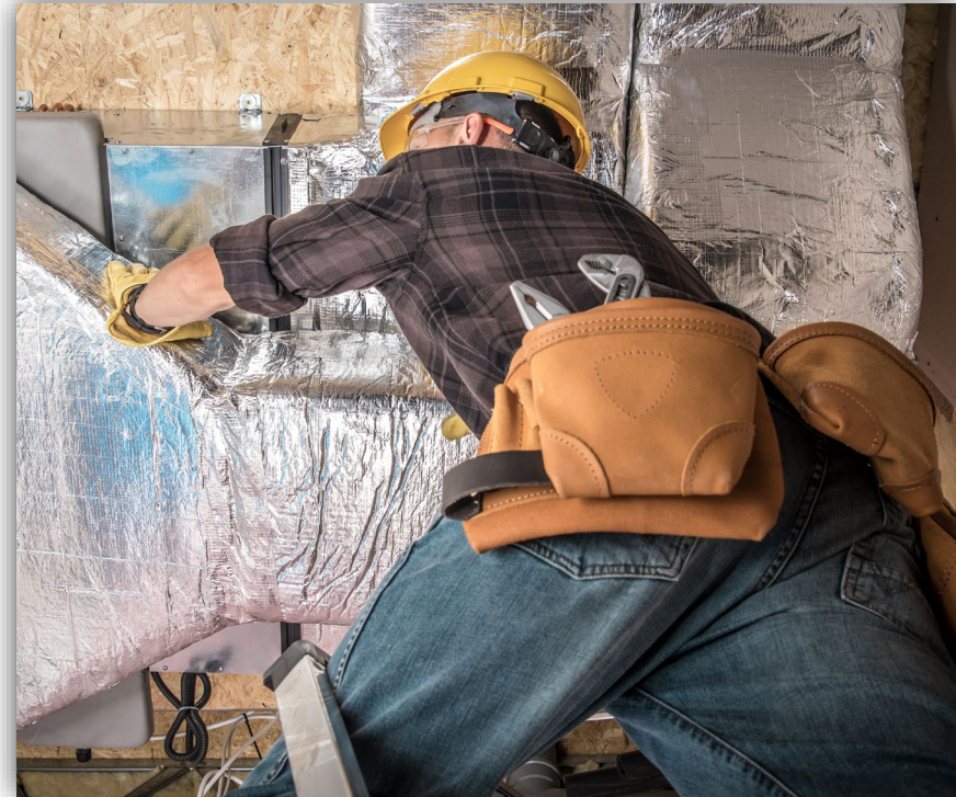
Image: Duct insulation installation
