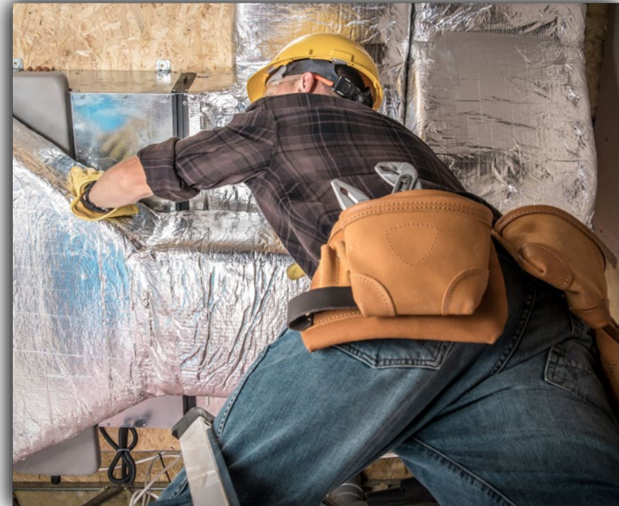
Image: Duct insulation
