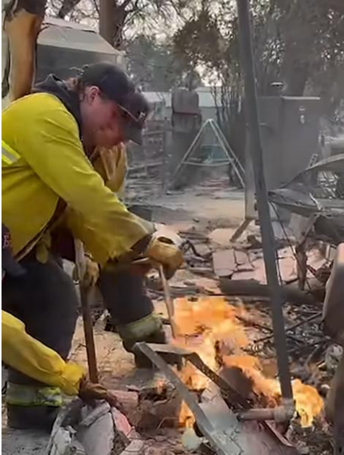
Firefighters excavate and shut off a natural gas service line in Altadena, January 2025
