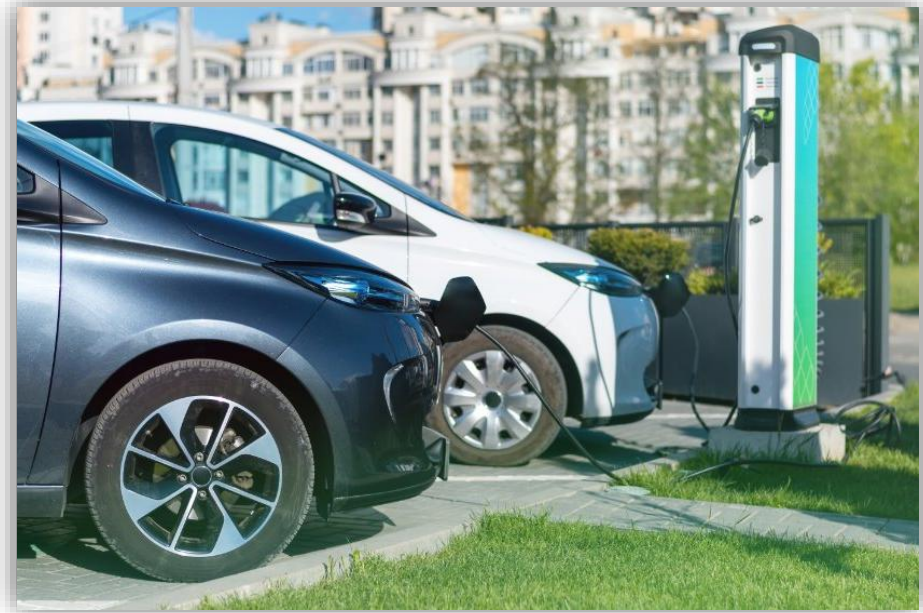
Electric Vehicle Infrastructure (EVI)
